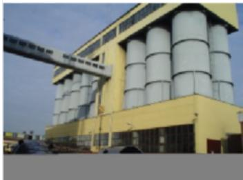
Our customer required continuous level measurement in several storage silos for carbon black which is used for the production of tyres. The particular challenge of this application is the extremely dusty environment, the low density of the carbon black and its stickiness.
