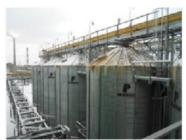
Our customer is one of the biggest supplier of plant oil in Sibiria. He requested a continuous level control for his storage silos containing grist. The storage contains of 10 slanting roof silos with each having a height of 14m. So far, the level was controlled manually by the employees. This kind of measurement is rather dangerous and also difficult in the winter.
