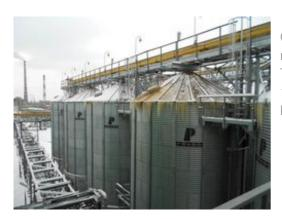
Our customer is one of the biggest supplier of plant oil in Sibiria. He requested a continuous level control for his storage silos containing grist. The storage contains of 10 slanting roof silos with each having a height of 14m. So far, the level was controlled manually by the employees. This kind of measurement is rather dangerous and also difficult in the winter.
