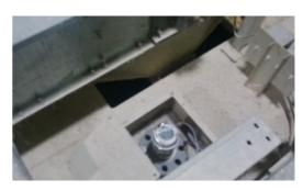
frequency of the sensor also provides an optimal echo confidence in this very dusty application. The standard air purge device for the lens antenna did not have to be activated.
