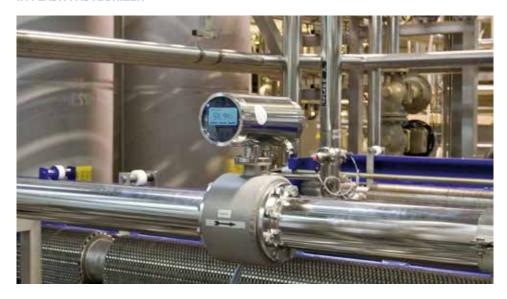
FLOW MEASUREMENT OF DEMINERALIZED WATER
